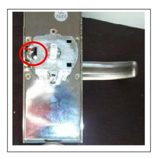
When the front mount is in place, hold the back mount rubber gasket against the back side of the door and place the back mount over the gasket and onto the stem protruding from the front mount.
